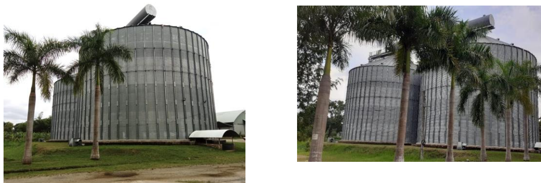
Figure 5.6: Maize Processing and Storage Complex of Five Star Grain Solution (Pvt) Ltd. in Siyabalanduwa, Monaragala District
